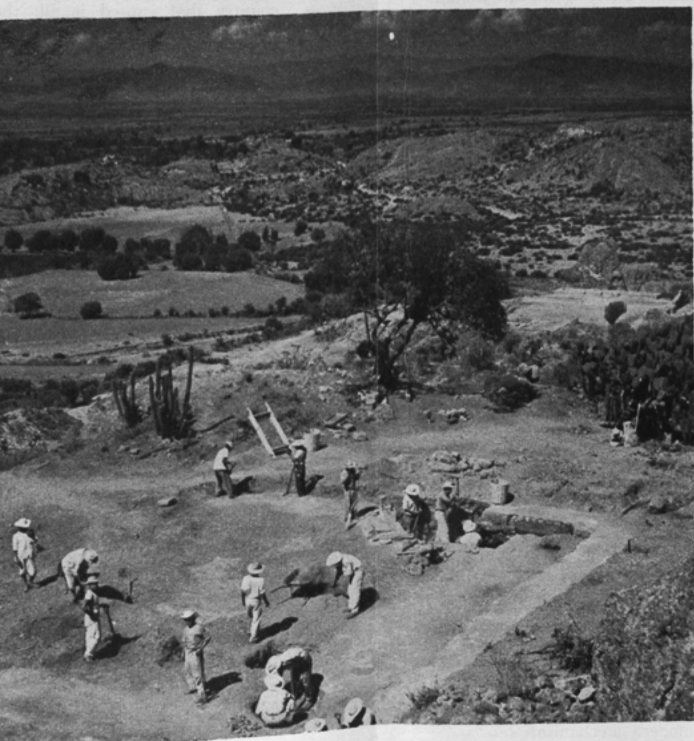
Workmen clear the large paved patio of an ancient house built over Tomb 28, apparently by those who broke into the tomb. In the upper right corner of the square patio is the pit leading to the tomb; in right background are the palaces of Yagul's Patio 1, cleared in previous seasons by MCC archeologists.
