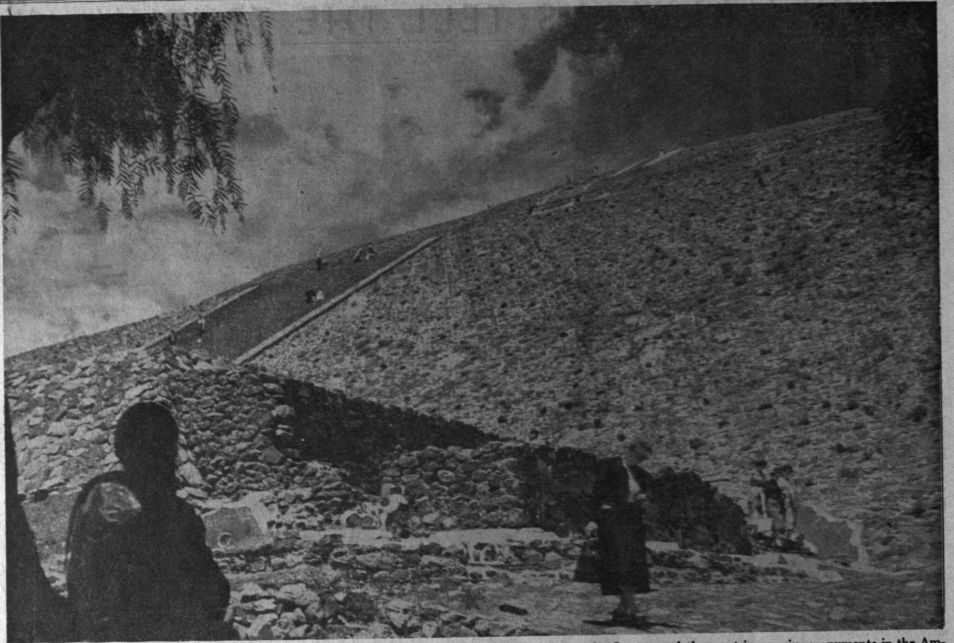
At Teotihuacan — “the place where all go to worship the gods” — is the Pyramid of the Sun, one of the most impressive monuments in the Americas. Almost 700 feet at the base, it rises to a height of over 200 feet. Built of adobe bricks from refuse of an earlier epoch, the exterior is faced with volcanic stone and covered with plaster, or pre-Spanish cement. (Photo by John Paddock).
