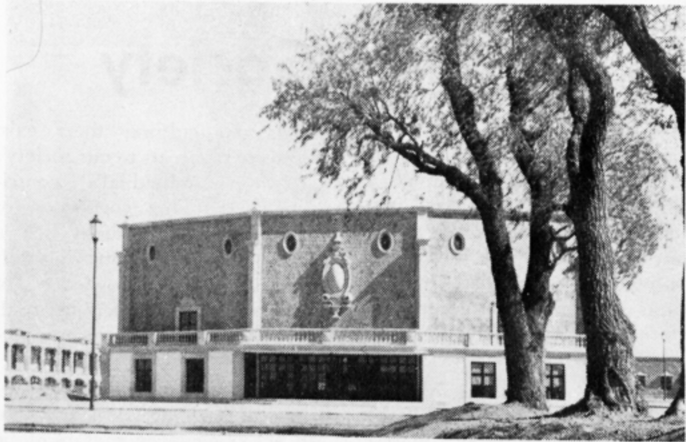
LECTURE CENTER —Brain center of the University, this building can be converted into a spacious hall for prominent guest lecturers, movie showings and theater productions. Its movable walls can also transform it into three lecture rooms.
