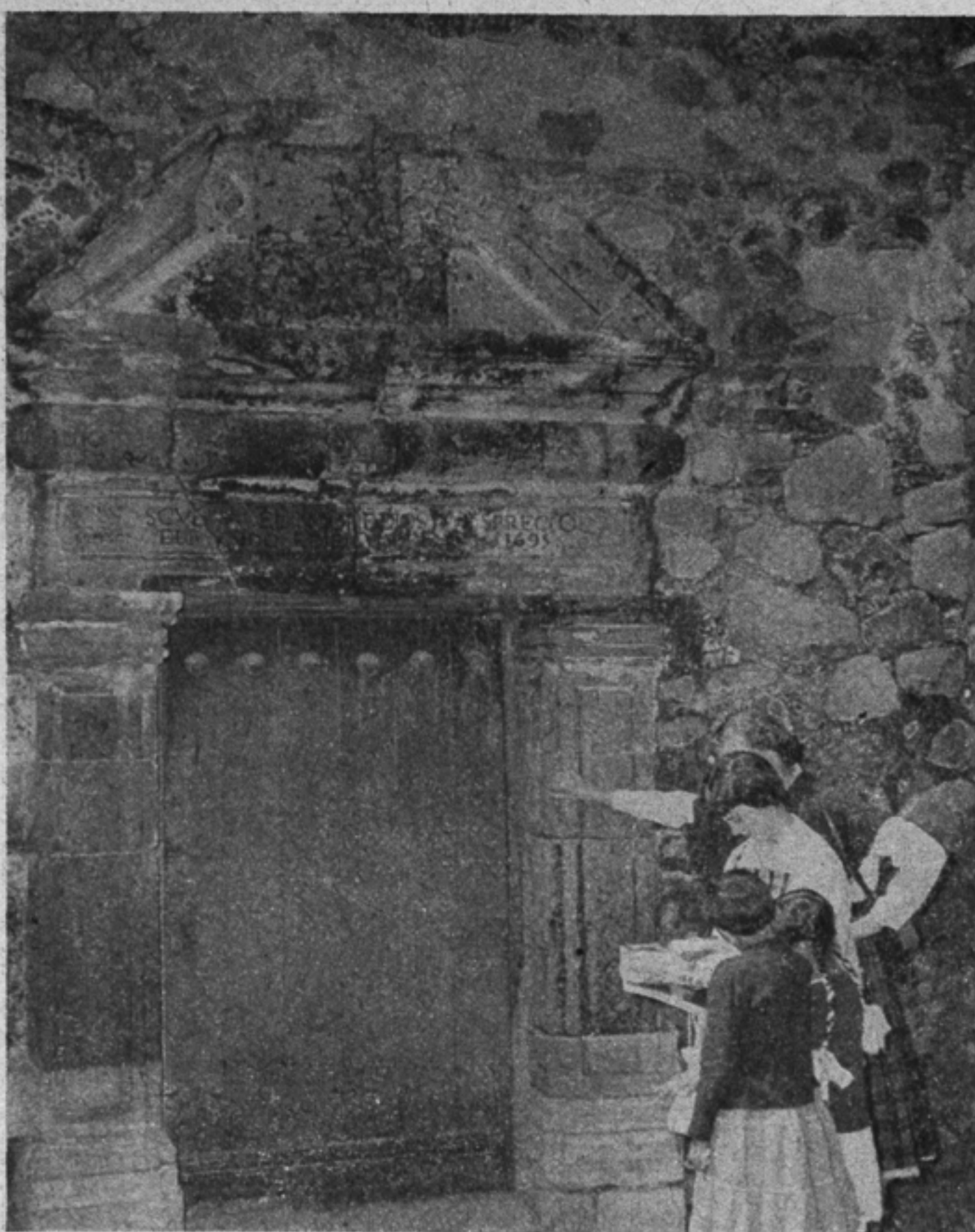
WHAT REMAINS of the chapel of Hospital del Amor de Dios y Desprecio del Mundo. Under the direction of "Tato Vasco", no one in the colony was allowed to labor more than six hours daily, beggars were unheard of, and the ownership of private property was forbidden.
