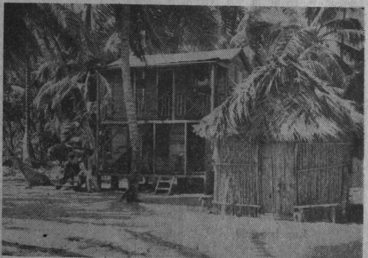
On the coast of British Honduras natives live in one house and cook in another. All wooden huts are built on piles for the sake of coolness and as protection against varmints. The cook hut in the foreground is made of palm leaves and cane stalks.
