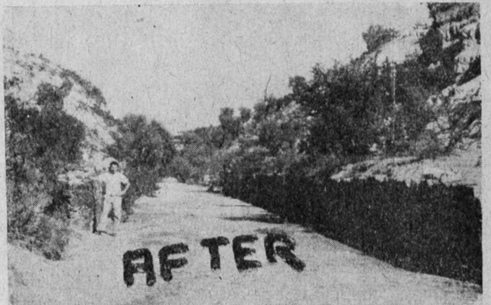
THE BEFORE AND AFTER photos above graphically show the dissipation of sixty years neglect. The before photo shows the canal constructed by Enrique Martínez to divert water from the Valley of Mexico. It took seven months to build and is five miles long. Ten thousand Indians died every mile of the way. The after photo shows the deterioration of the system and the complete lack of water.
