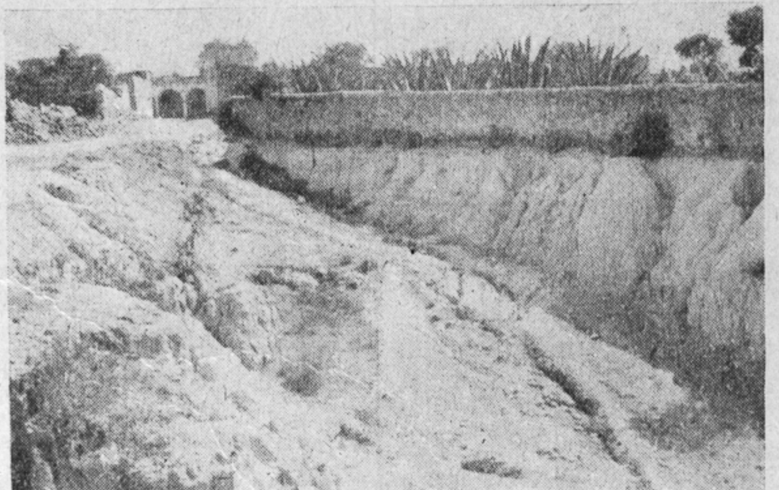
DISAPPEARING CITIES. Not only are the natural resources of the land ravished by the rains, but man's work itself crumbles before their onslaught. The above photo shows what is happening to the capital city of the township of Huehuetoca. The gully has moved through the outskirts of the town and is now eating across the main street into the heart of the city.
