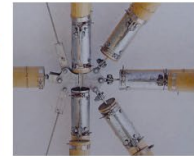
Bamboo in construction with bespoke nodes
