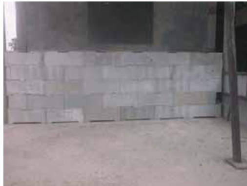
Figura 19: Blocks de concreto autoalineables
