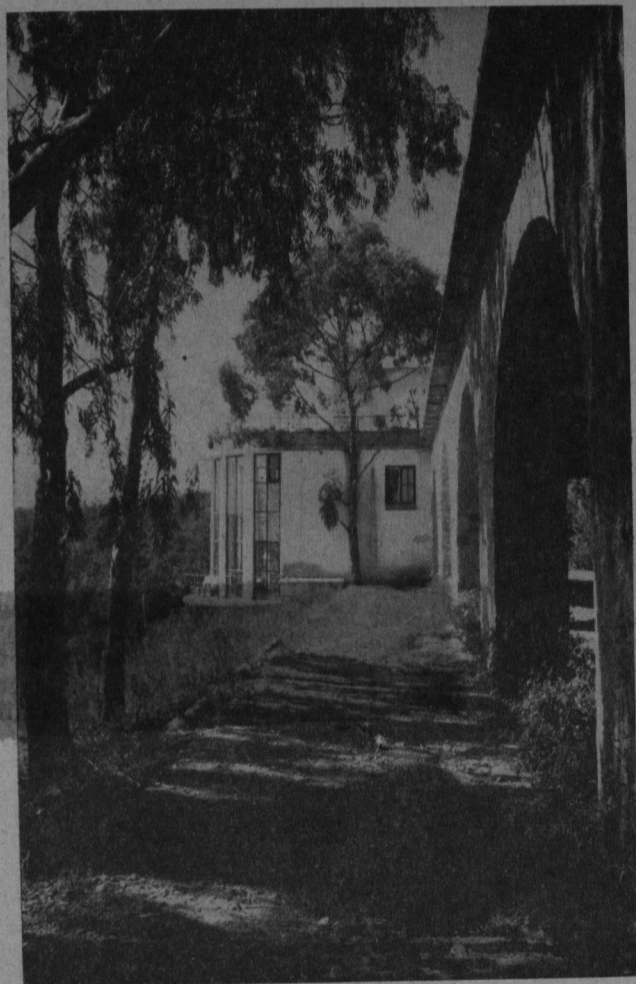
SUNLIGHT STREAMS INTO THE CLASSROOMS.
